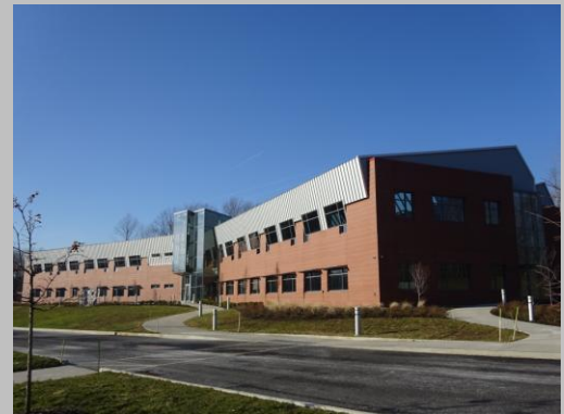
The Advanced Manufacturing Project was another one million plus project which consisted of large custom stainless gutters, metal roof and wall panels and a 30 year EPDM roof system
